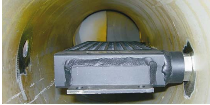
Remove air cooler in air duct
