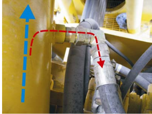
Air compressor inlet air from fitting in air duct
